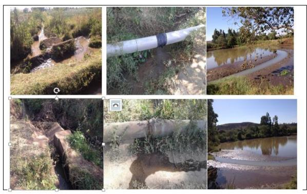
Figure 10. Irrigation water conveyance systems damaged canals (left) broken PVC (middle) and pond filled with sediments (right) (Source: own picture 2017)
